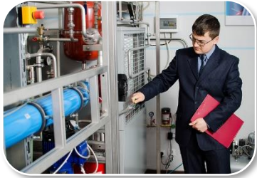
Automation and Control
